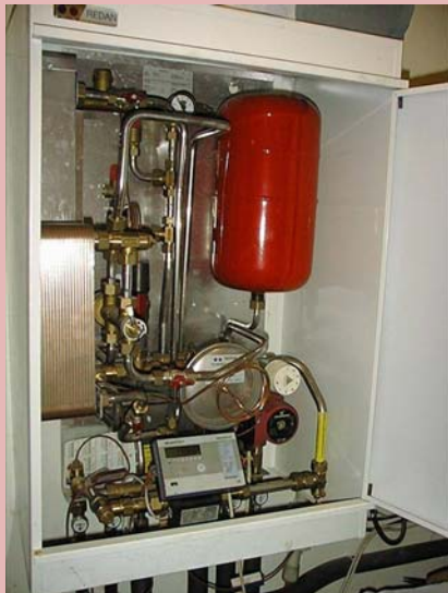
Above: A typical heat exchange unit
