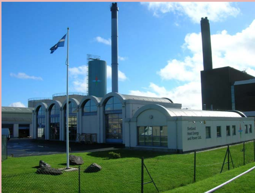
Above: The SHEPL offices and peak load boiler station. The large silo at the rear is the thermal store. Behind the plant is the Lerwick Oil Fired Power Station
